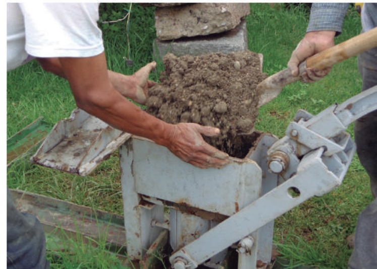
Fills molds and apply pressure ③
