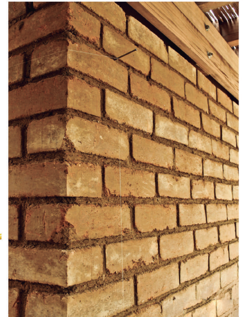
Finished walls ⑧
