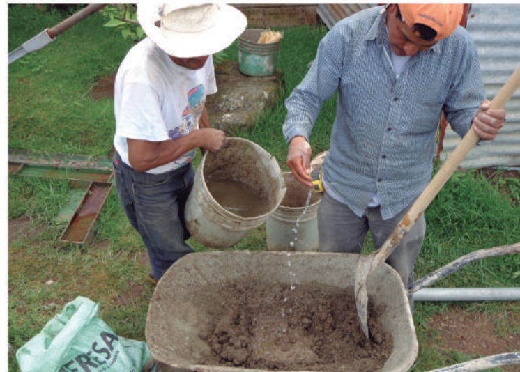
Mixture of cement, water and earth ②
