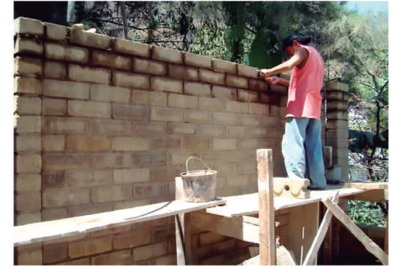
Construction of walls ⑦
